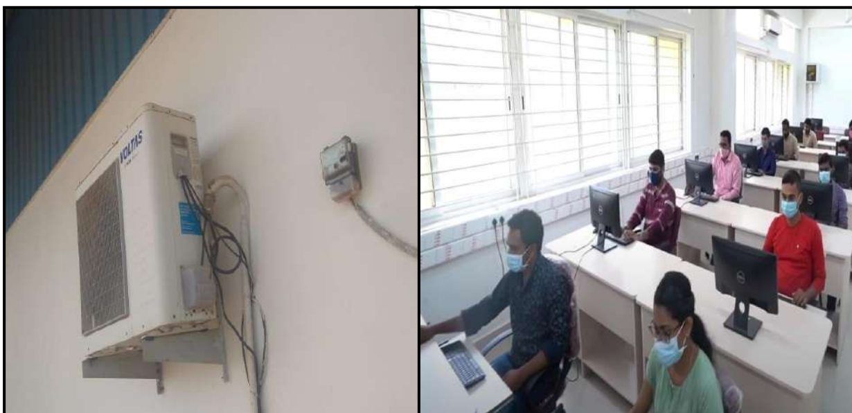
Ventilation & Exhaust Facility at CUTN Campus, Thiruvarur, Tamil Nadu
