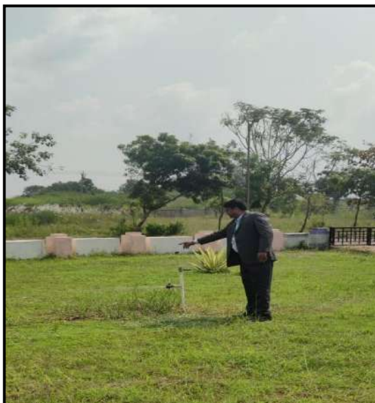
Irrigation Facilities in CUTN Campus, Thiruvapur, Tamil Nadu
