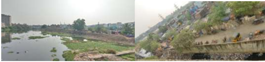
Fig. 9: Adyar river, Saidapet and Buckingham canal, Raja Annamalai puram, Chennai (Source: taken by author)
